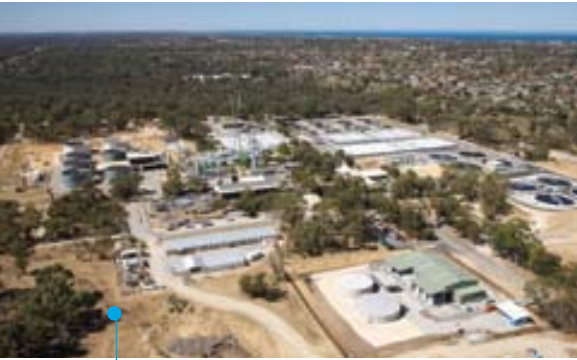
Groundwater Replenishment Trial, WA (courtesy of WA Water Corporation)
